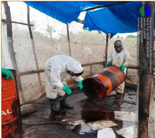
Inside the “Workshop Area” – sorbent booms lining with layered plastic tarp to contain oil during cleaning
