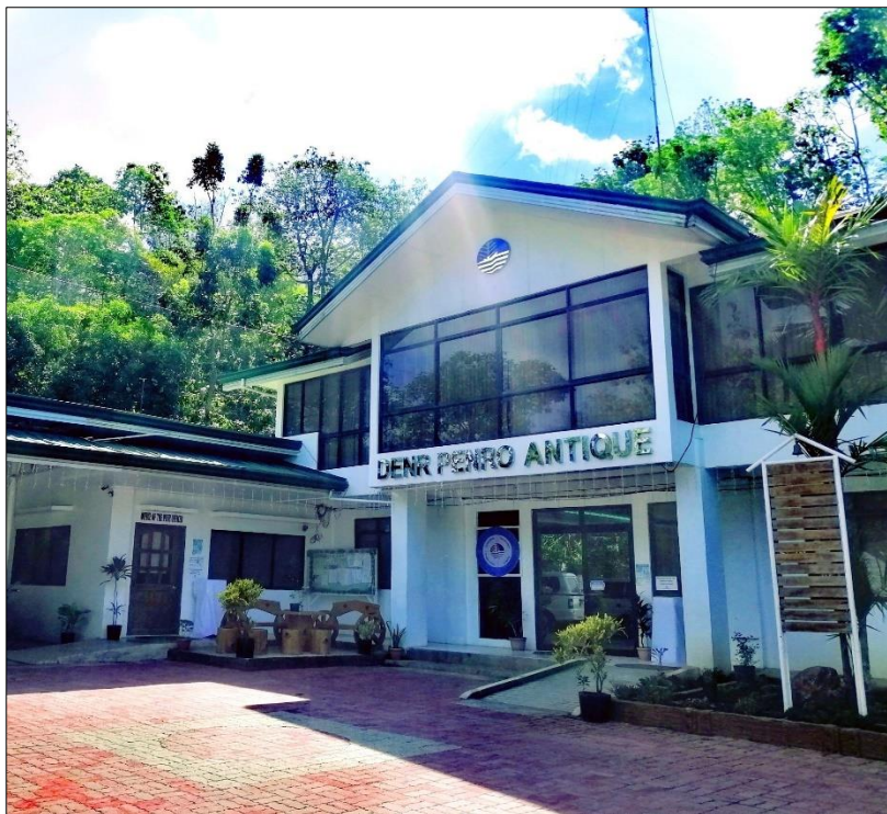
The current PENRO Antique Office Building
