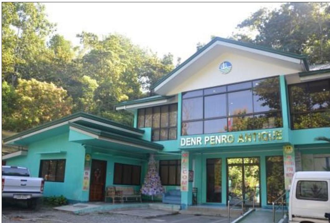
The renovated PENRO Antique Office Building in the year 2013
