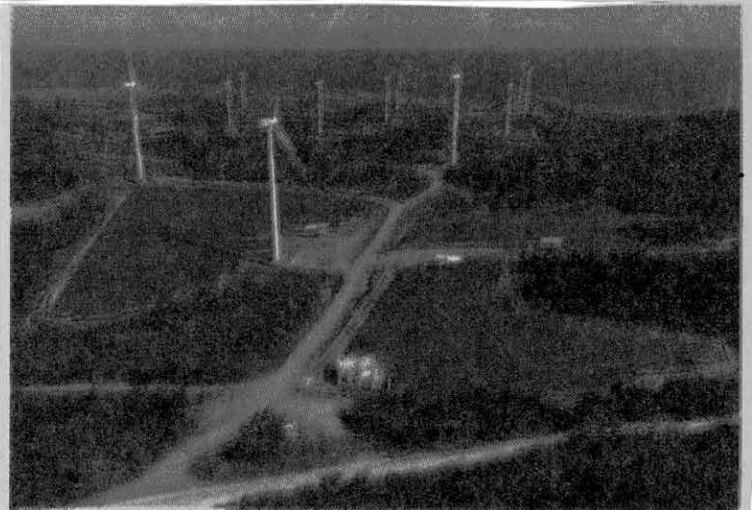
EDC's 150MW wind and 6.8MW solar farm is the first combined RE facility in the country.
